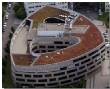
Photovoltaics, ZSW Stuttgart
